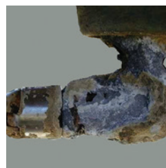
Unprotected sail drive
